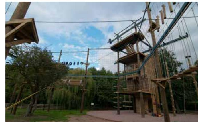
The high ropes adventure course will be a series of obstacles supported on wires that in turn are suspended between timber posts. As the cable system does not need a large steel structure to support itself the course will have very little visual impact particularly as it will be sandwiched between the existing and newly planted trees to the south and trees and range netting to the north.
